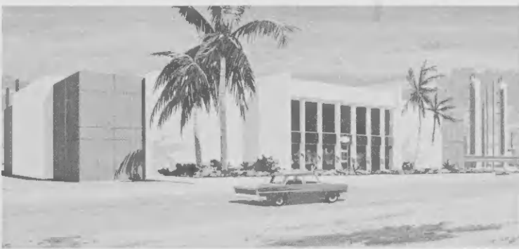
The Refining Controlhouse now being expanded contains six process computers to control the operations of practically all refinery units. It's scheduled for completion this month.
